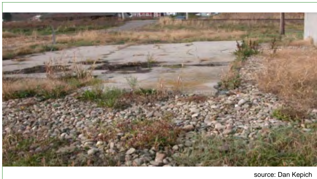
Figure 2-2-6 Sloped, Concrete Gravel Pad for Equipment Cleaning
